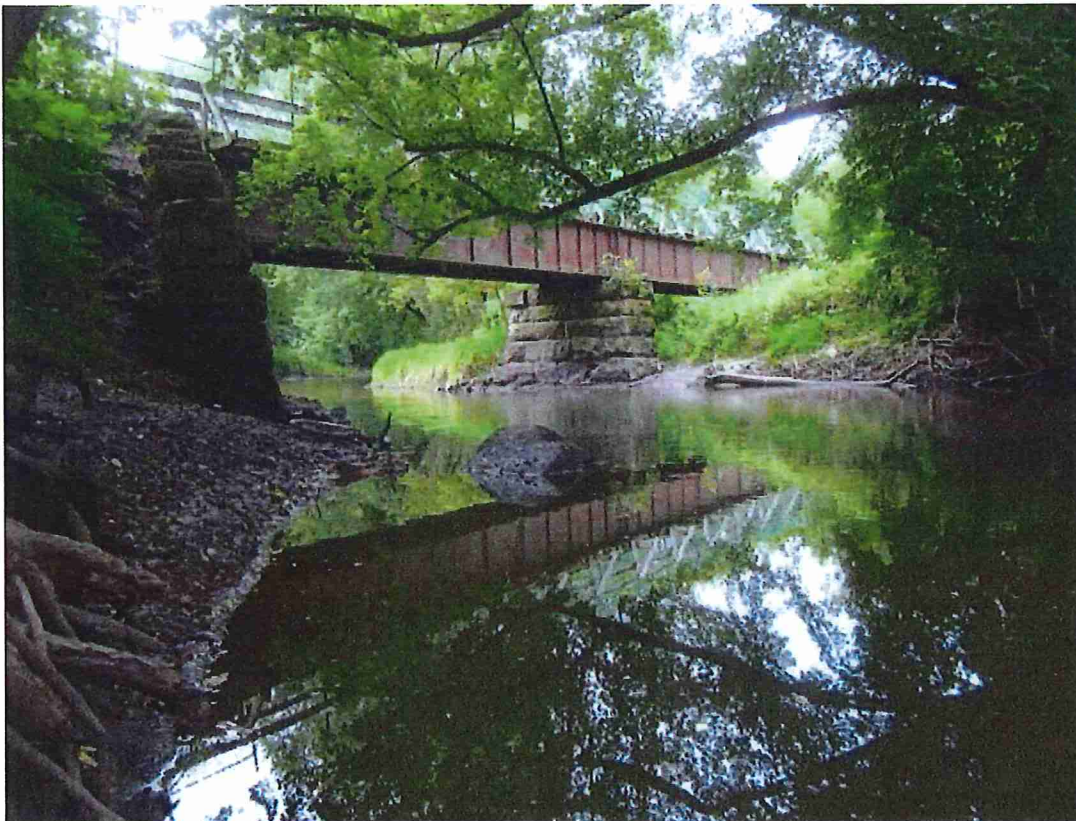
Existing Steel Plate Girder Spans (Looking NW)
