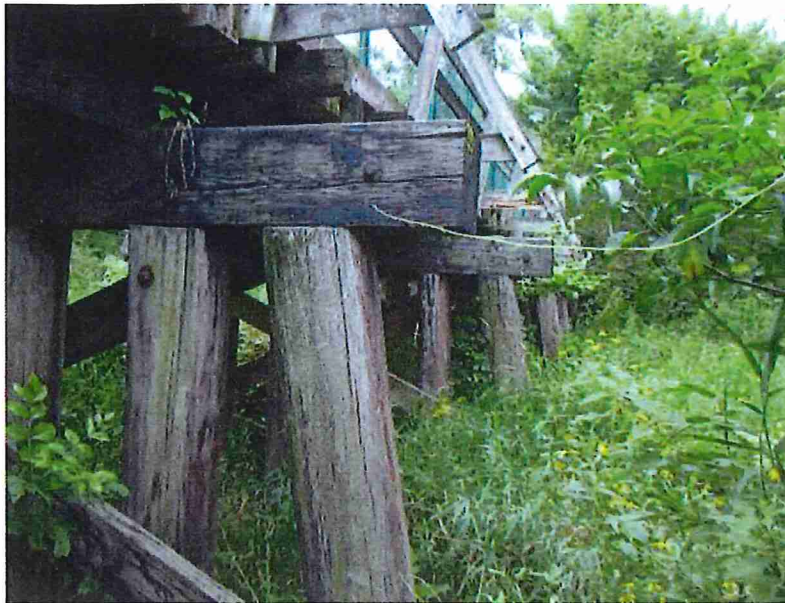
Existing Timber Beam Spans (Looking NW)
