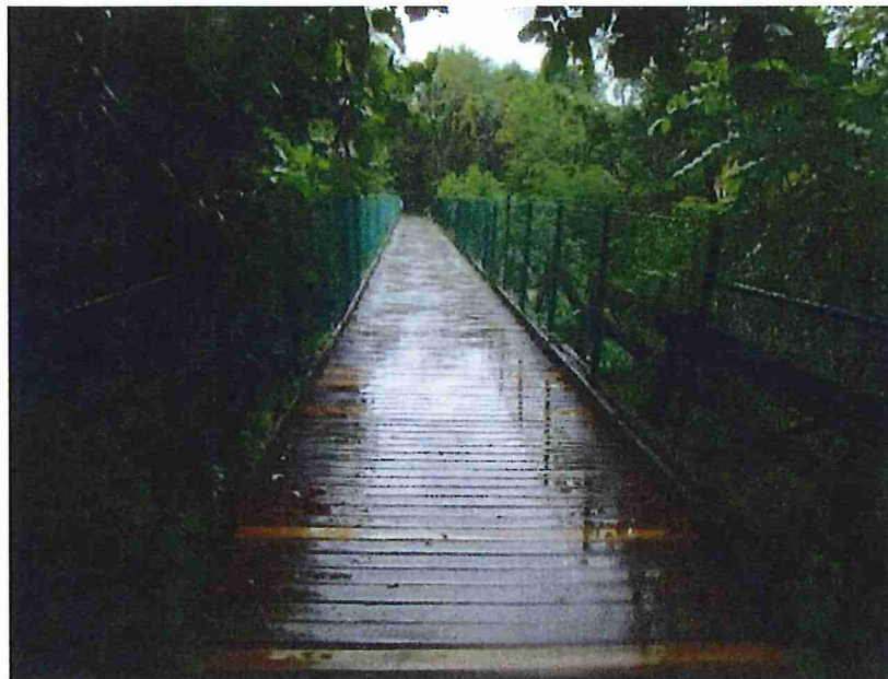
Existing Timber Deck (looking South)
