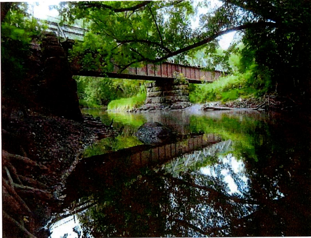
Existing Steel Plate Girder Spans (Looking NW)
