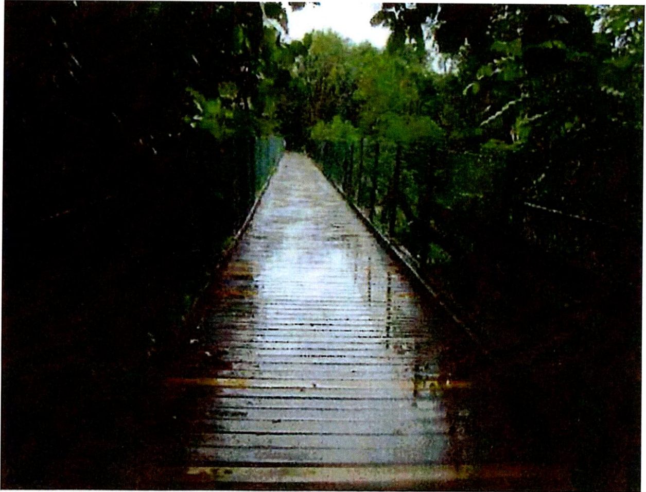
Existing Timber Deck (looking South)
