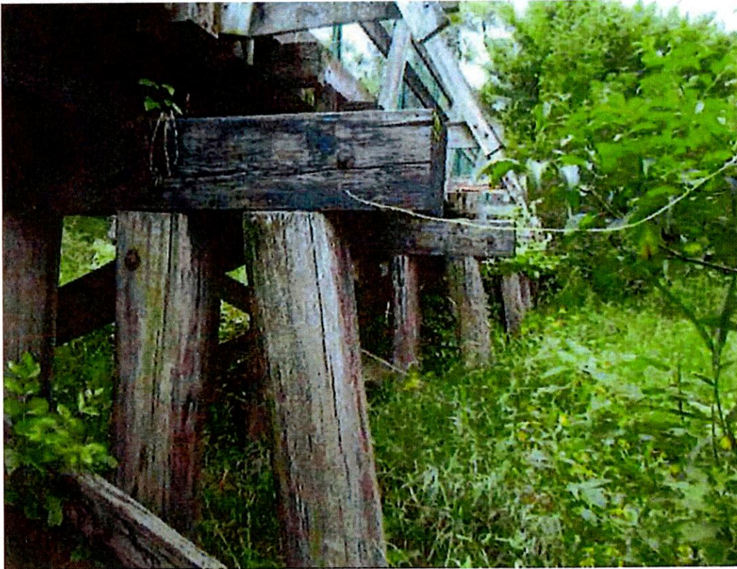
Existing Timber Beam Spans (Looking NW)
